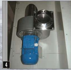
4 Air cooling extractor
